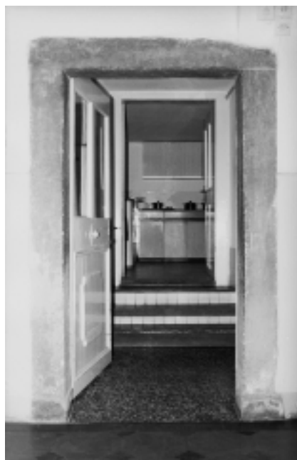
Kameni okvir vrata koja povezuju dva hodnika u prizemlju pročelnog krila kurije. Vidi se povišenje podne razine prostorije uz pročelje koje je nastalo naknadno; snimio T. Križić Stone door frame connecting two corridors on the ground floor of the main wing. Noticeable the raised floor level of the room along the facade which was added later (photo: T. Križić)
