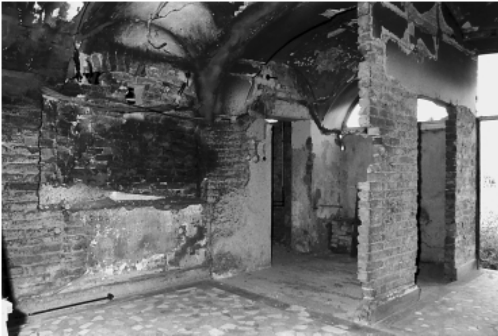
Županijska palača, detalj hodnika u prizemlju (foto: Milan Drnić) County Palace, detail of a ground-floor corridor (photo by Milan Drnić)
