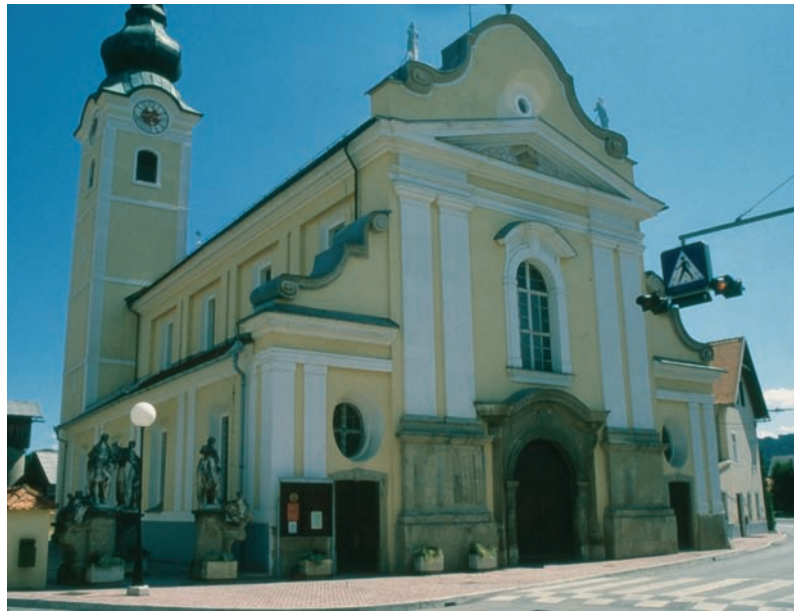
Petrovče, Crkva sv. Marije, pročelje (foto: B. Badovinac) Petrovče, church of St Mary, façade
