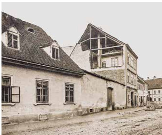
5. Dvokatna ugrađena najamna kuća u današnjoj Masarykovoju ulici nakon potresa 1880. One-storey built-in rental house in today's Masarykova Street after the earthquake of 1880
