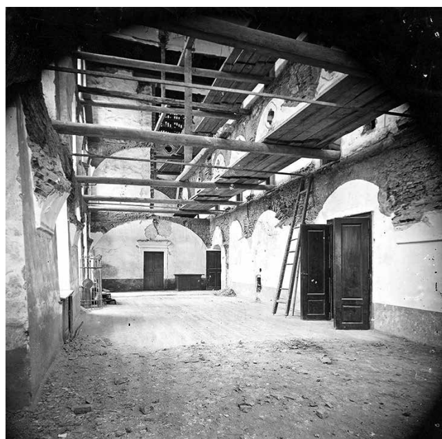
6. Srušeni svodovi nakon potresa 1880. Demolished vaults after the earthquake of 1880
